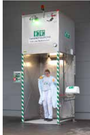
Tanknotduschen Tank safety showers
